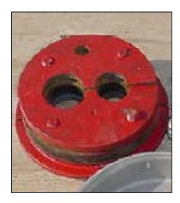
The other type of seal is an overlapping exterior sanitary well seal, illustrated in Exhibit 4.3. It is commonly used in outdoor applications with submersible pumps and pitless adapter units. The vent is under the lip, and gasket material seals all openings around the casing and conduit.
