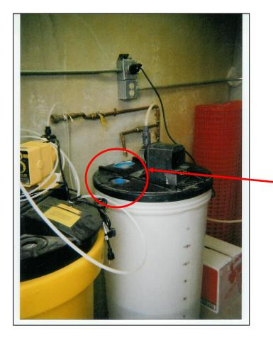
Air gap between water feed and chlorine solution
