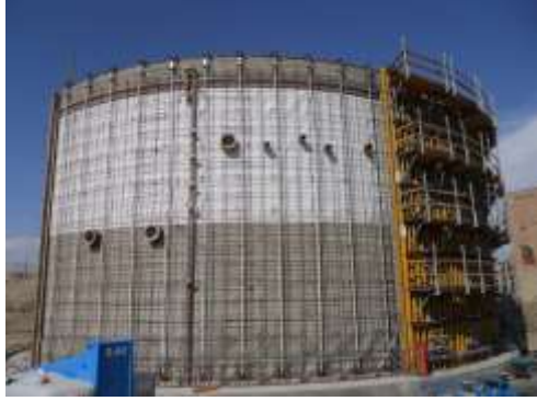
Interior Lining – Wall Penetrations
