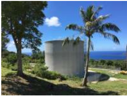
300,000 Gallon Water Storage Reservoir Saipan
