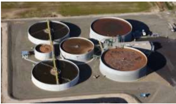
Livingston, California (2) 2.3 MG Aerobic Digesters (2) 1.3 MG Clarifiers 1.0 MG Anoxic Reactor 0.25 MG Aerobic Reactor
