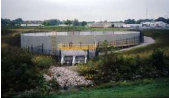
Indianapolis, Indiana | 1.35 MG storm water tank
