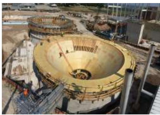
Structurally Supported Conical Floor
