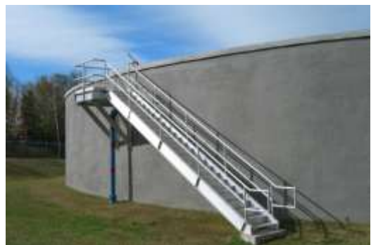
stairs and landing
