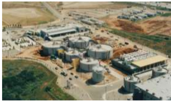
San Diego, California two 0.5 MG receiving tanks two 1.4 MG anaerobic digesters three 3.1 MG anaerobic digesters
