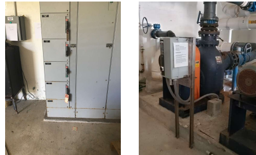
Mount the Control Panel Threshold higher than the pump pedestal. & all the pumps are over-sized.
